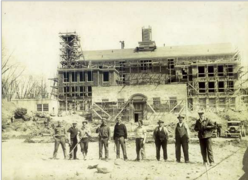
First junior high school under construction in the 1930s, viewed from the rear
